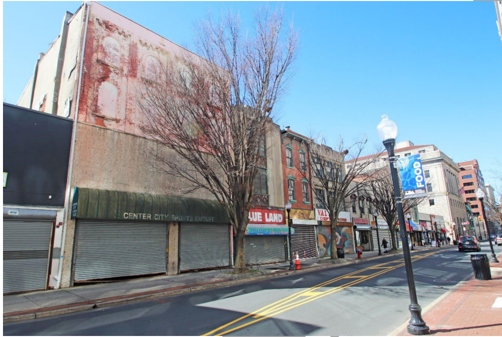
Photo 3 - East State Street, south side, looking southeast from the midpoint of the block. The four-story building at far left is 27-29 E. State Street (#12).
