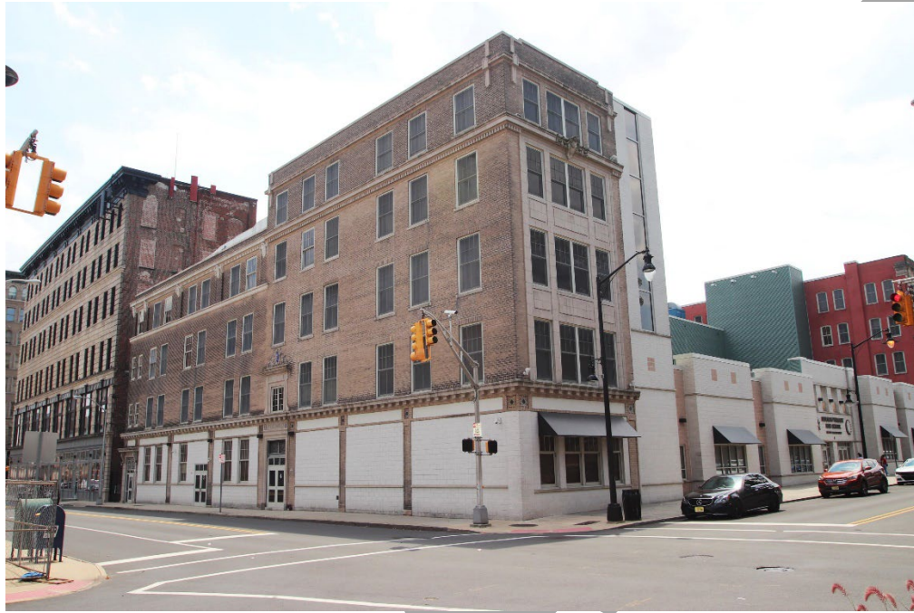
Photo 19 – The Fitzcharles Building at 147 E. Hanover Street (#51c), looking southwest.
