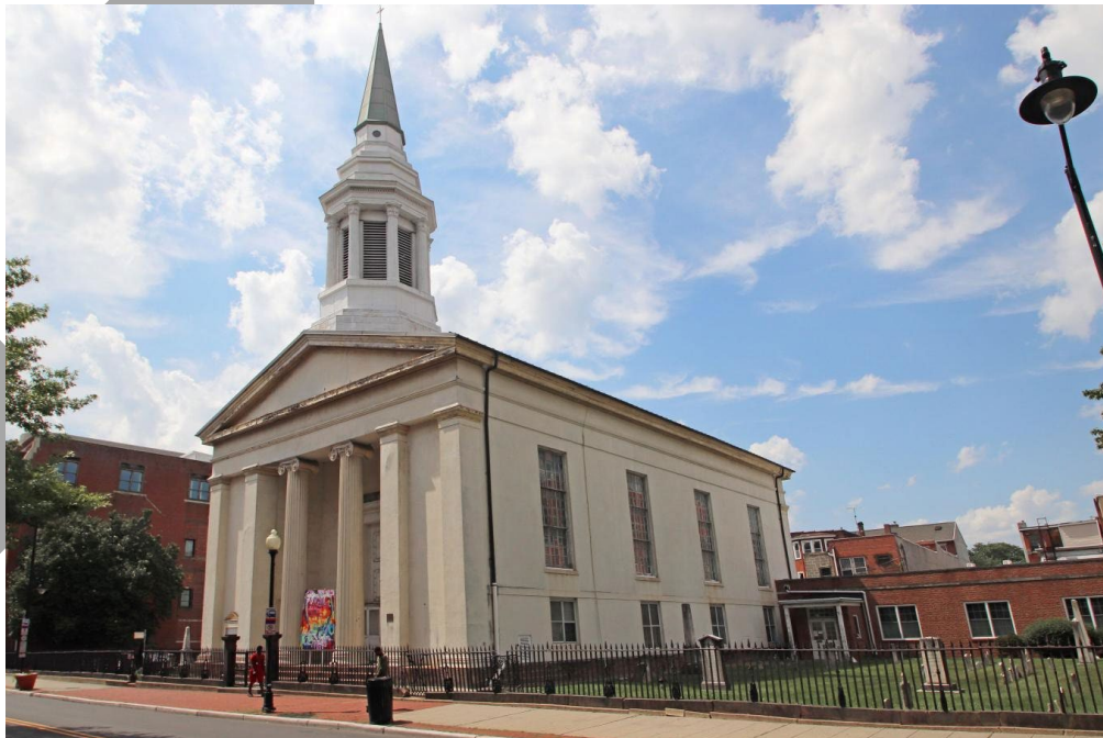
Photo 8 – The First Presbyterian Church at 120 E. State Street (#32), looking northwest.
