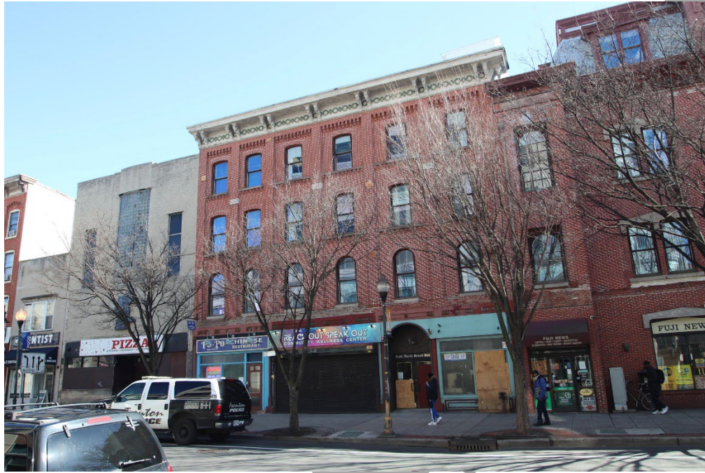
Photo 13 – North Broad Street, west side, looking northeast. 4-8 North Broad Street (#38b) is at center.
