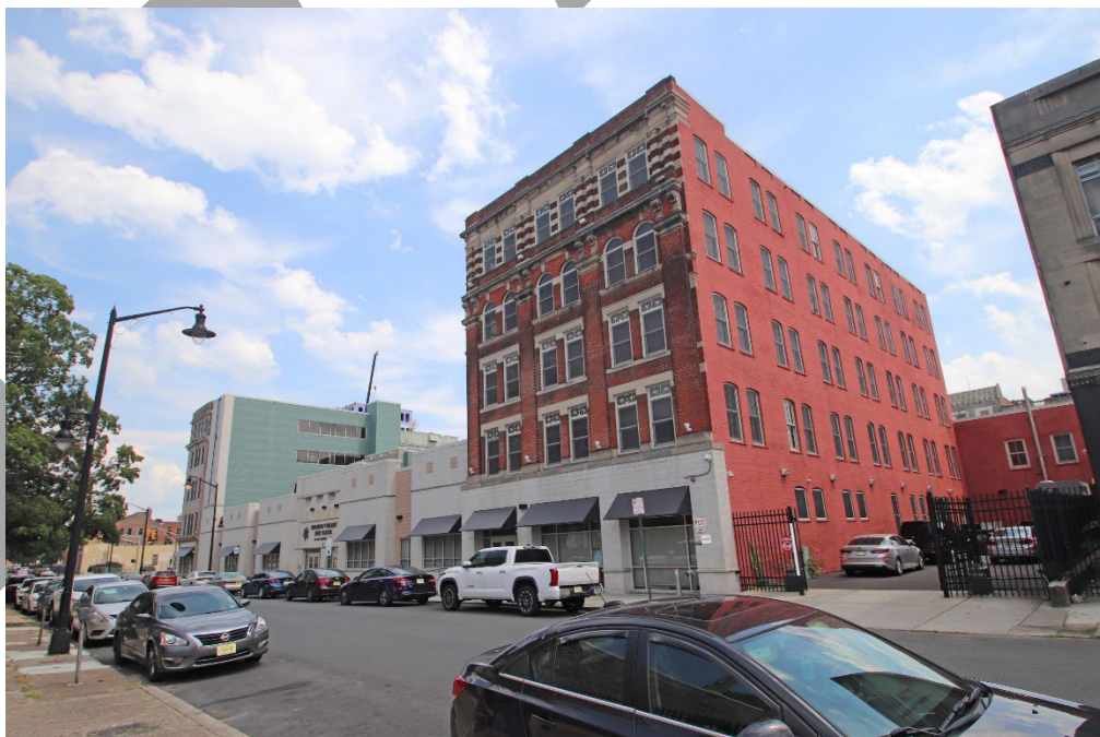
Photo 18 – The Trenton State Gazette Building at 127-129 E. Hanover Street (#51a), looking southeast.
