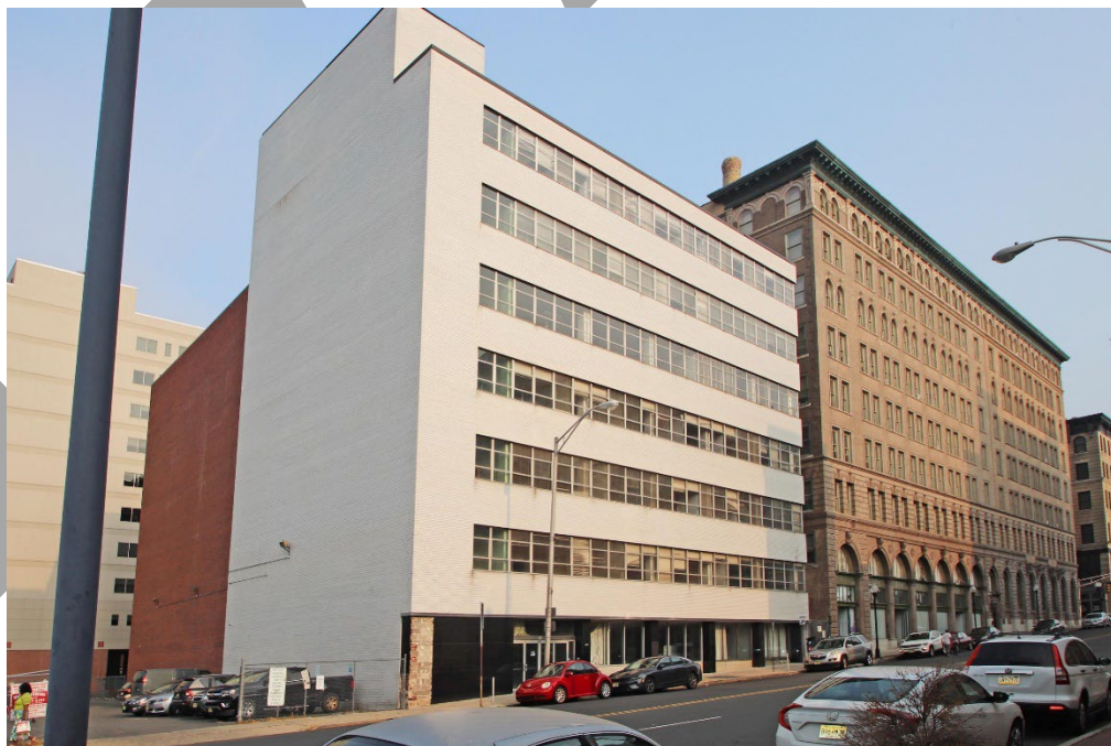
Photo 20 – South Montgomery Street, west side, looking northeast. In the foreground is the New Jersey Division of Motor Vehicles Building at 25 S. Montgomery Street (#52).
