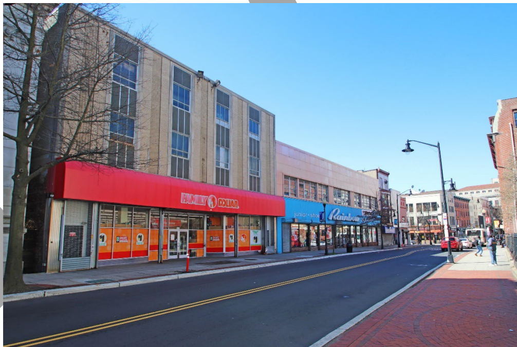
Photo 6 – The F.W. Woolworth Store at 117-121 E. State Street (#25) and the S.S. Kresge Store at 109-115 E. State Street (#24), looking southwest from the north side of State Street.
