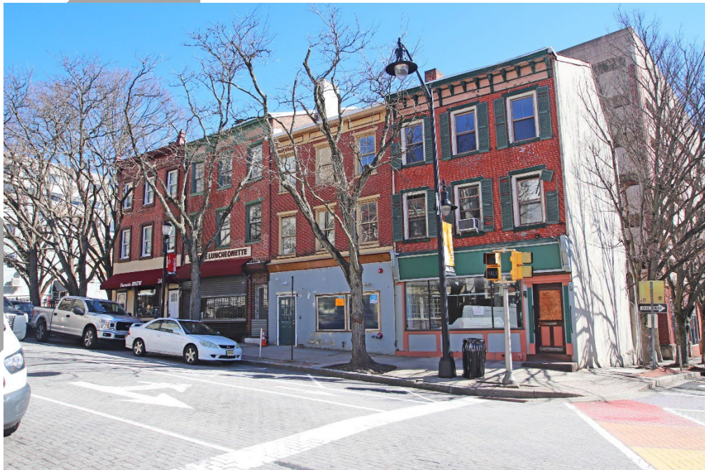
Photo 22 – 24-30 S. Warren Street (#57-60), looking northeast.
